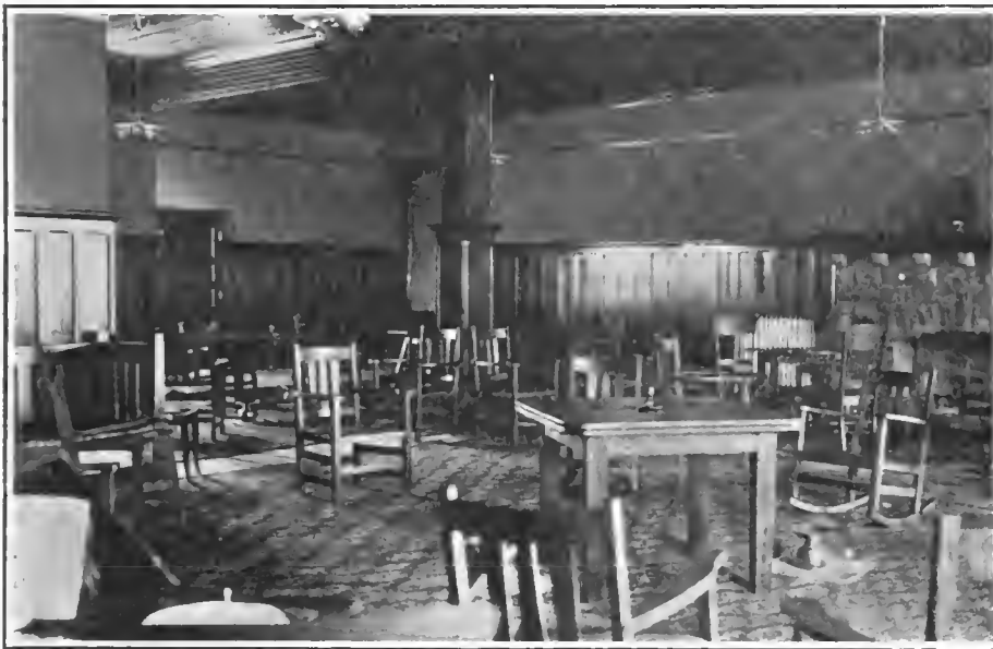
ASSEMBLY ROOM IN THE NEW QUARTERS OF THE BUFFALO AUTOMOBILE CLUB
